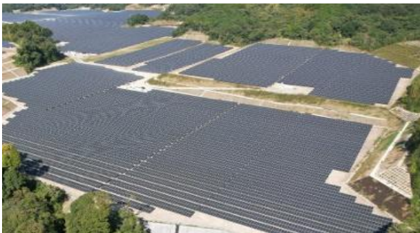
Panoramic view of solar power plant
