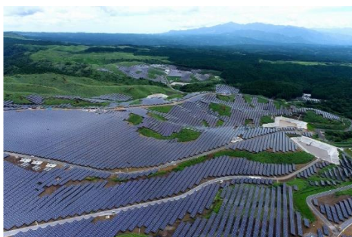
JRE Yamato Takamori 1 Solar Power Plant
