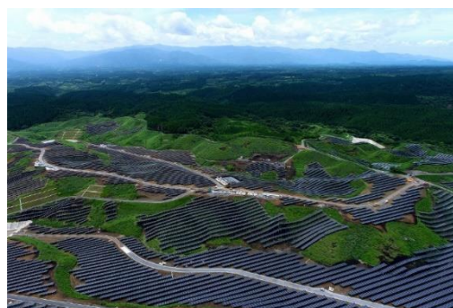
JRE Yamato Takamori 2 Solar Power Plant
