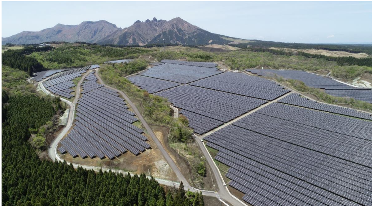
JRE Aso Takamori Solar Power Plant
